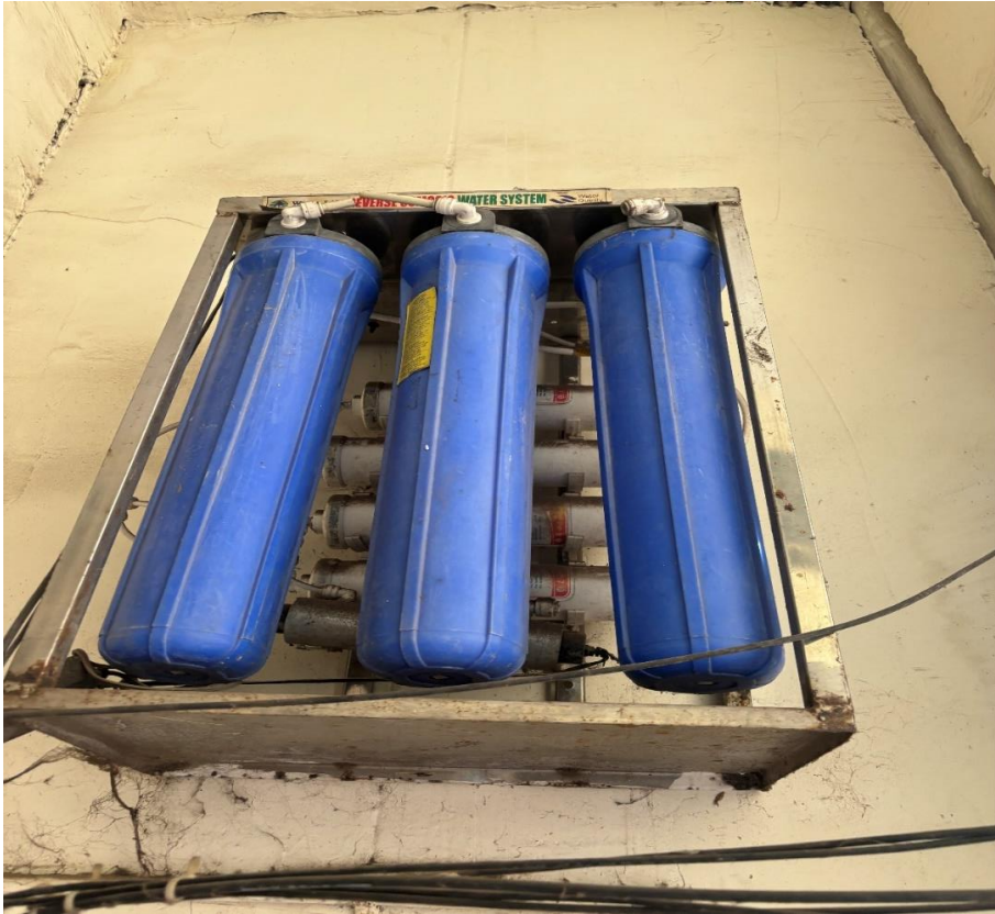
INSTALATION OF RO WATER PLANT BY OUR ALUMNI
